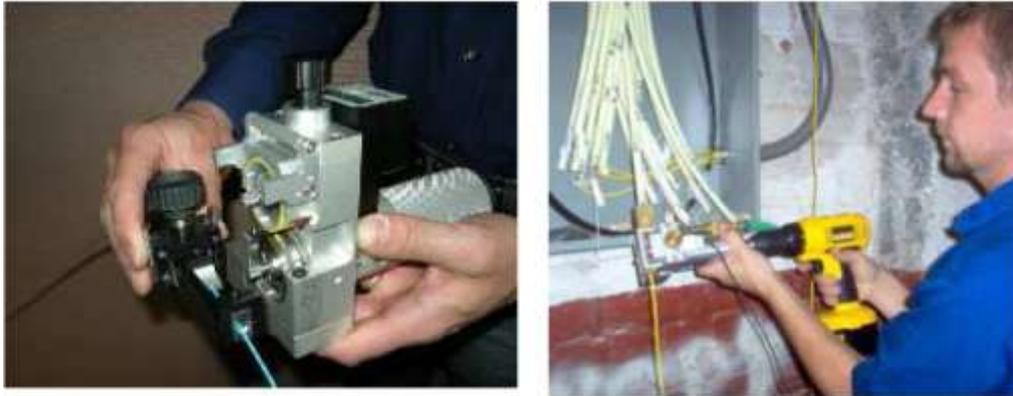
**Figure 8:** Field trial, installing the cartridge, jetting from MDU Terminal
